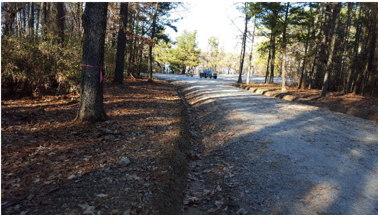
PHOTO 6 HELLER'S CREEK PUBLIC ACCESS AREA
