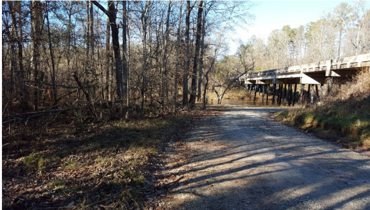
PHOTO 8 ENOREE RIVER BRIDGE INFORMAL ACCESS AREA
